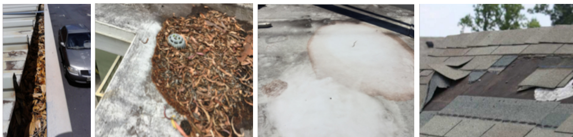
A few of the top common roof failure points include clogged gutters and downspouts, poor drainage, punctures, and missing shingles.
