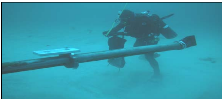
Figure IV.1. Diver working on off-shore conduit facilities that shield fiber cables from surf zone damage and protect coral reef habitats from potential harm due to cable trenching or drift.
