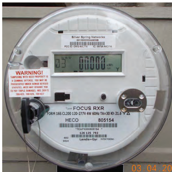
Figure 1. Photograph of the Landis+Gyr smart meter deployed by Hawaiian Electric Company .
