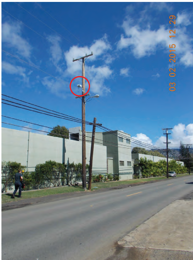
Figure 4. Relay device installed on an electric power pole at site 11 (see red circle). Measurements were performed along the edge of the street on both sides of the power pole.
