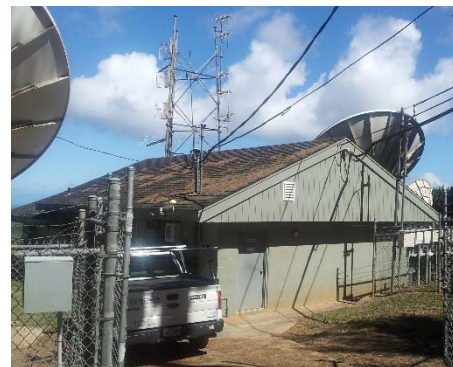
Figure 2: Headend Building at Kalaheo
