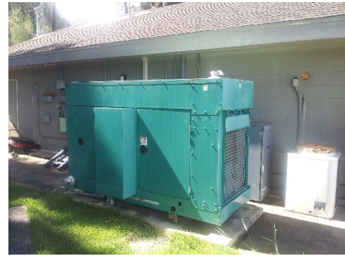
Figure 3: Generator at Kalaheo Headend
